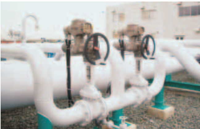
SAEXC multi-turn actuators with AMEXC controls within the kerosene distribution system of Chubu airport in Japan.
