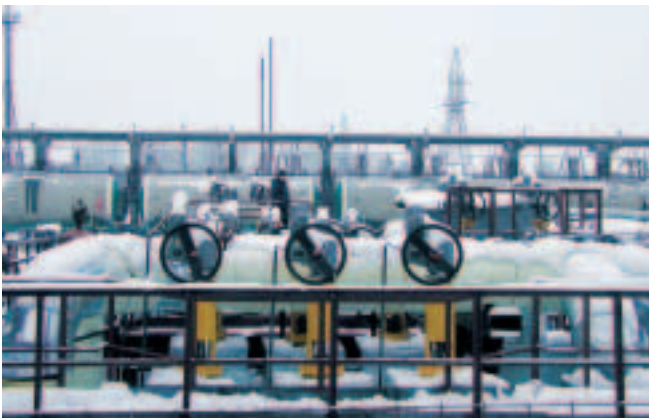
Extreme weather conditions at the polar sea. SA multi-turn actuators with AUMA MATIC in a tank farm near Arkhangelsk in the North of Russia.
